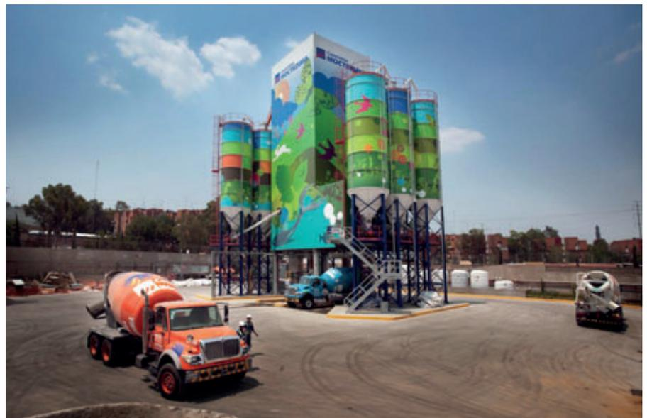
*The tower batching plant is equipped with the latest generation systems (including a 2.5 m<sup>3</sup> concrete mixer)*
