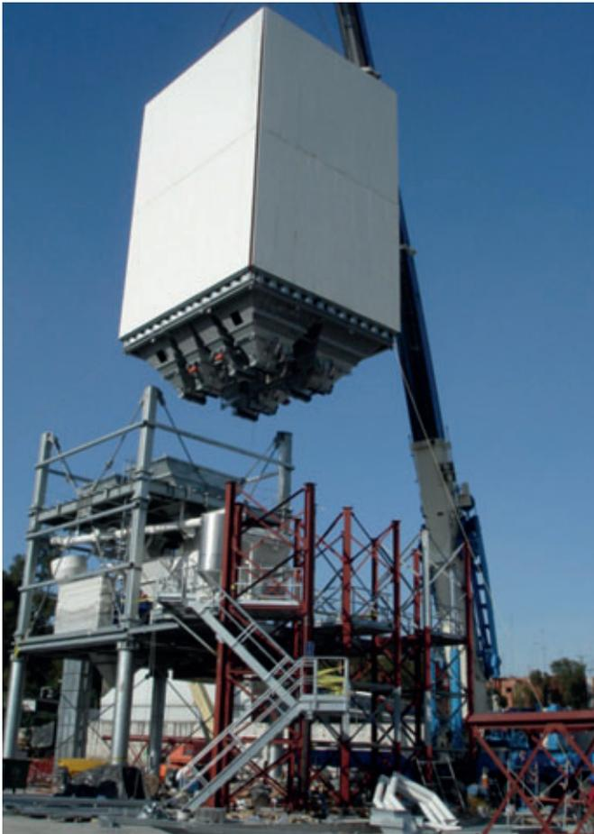
*Aggregates storage system with 8 hoppers – total capacity of 600 m<sup>3</sup>*
