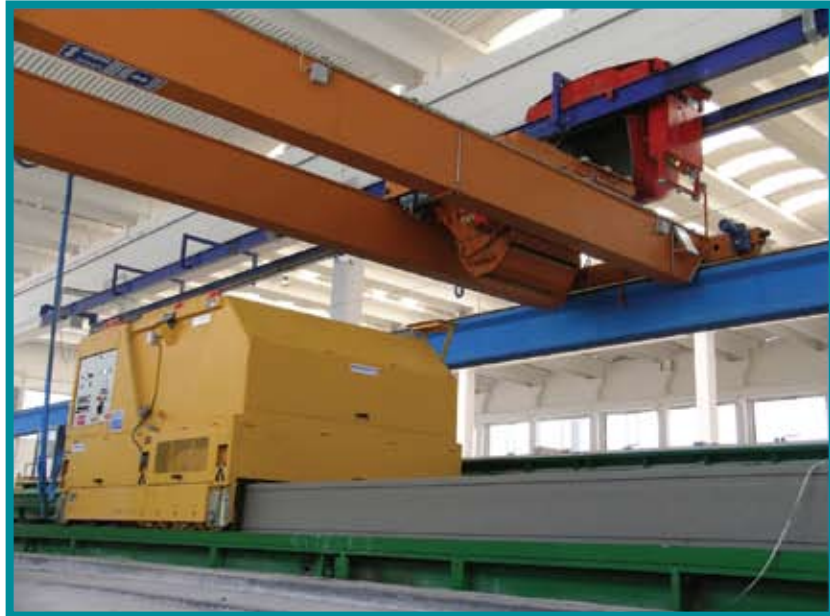
CONCRETE DISCHARGE FROM OVERHEAD FLYING BUCKET TO CASTING BUCKET
