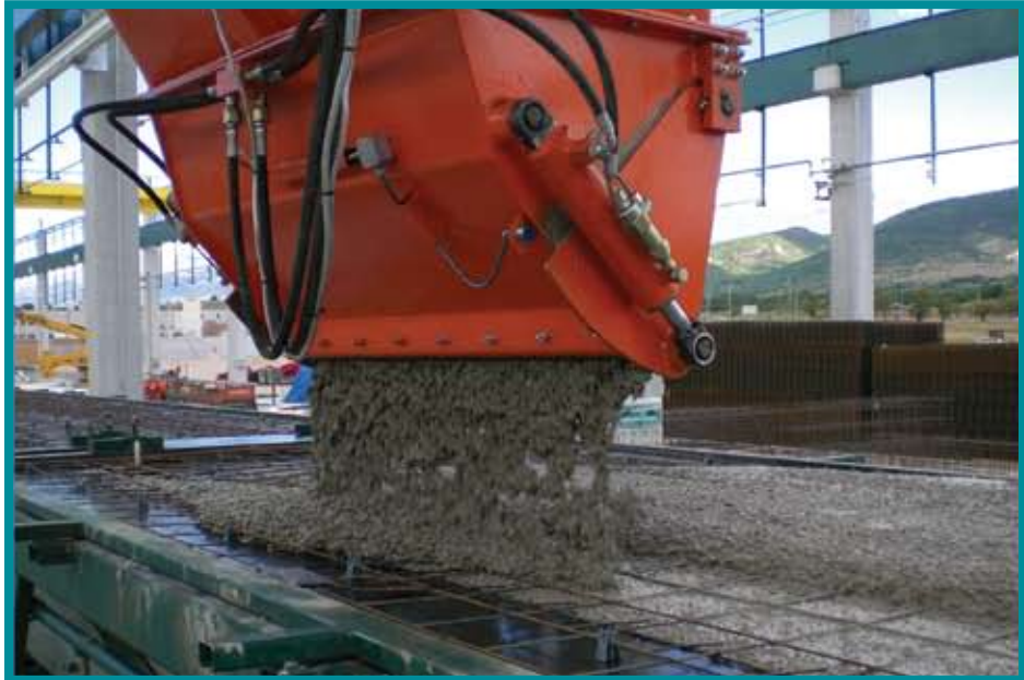
CASTING BUCKET IN OPERATION
